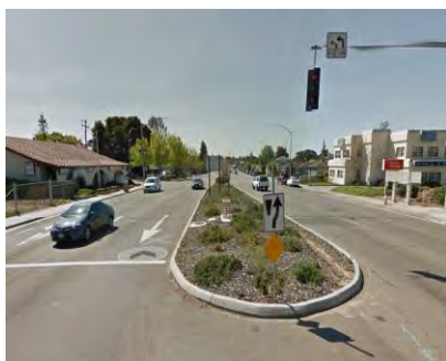
Redwood Road looking south from the I-580 undercrossing
