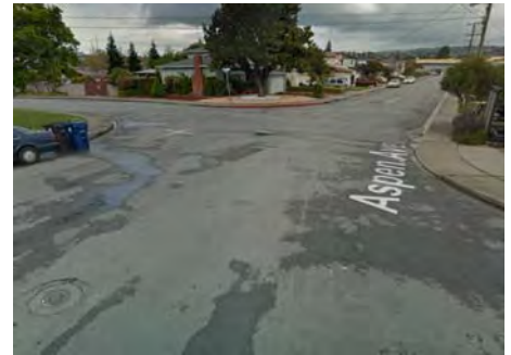
Intersection of Aspen Avenue and Pine Street looking West along Pine Street
